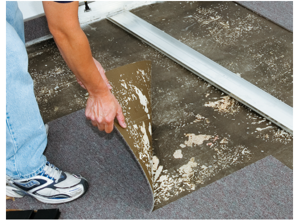
Remove carpet tiles to expose concrete
